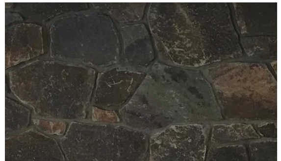
Example of a client-supplied fire box lining
