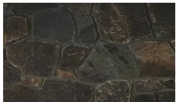
Example of a client -supplied fire box lining
