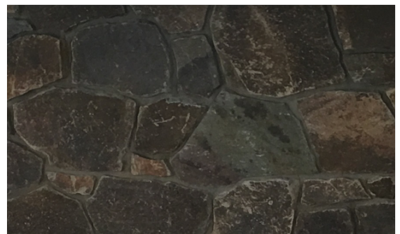
Example of a client-supplied fire box lining
